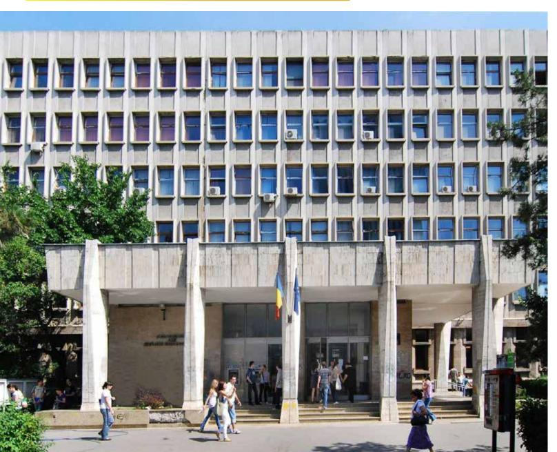
The current building which was designed and built in the 60's, will include the rehabilitation of the supporting structure, thermal insulation for the exterior and floors, upgrade of the ventilation and sanitary installations, reconstruction of the inner and outer finishings and replacement of the elevators. Also, the building will be equipped with solar panels, providing a renewable source of energy.
